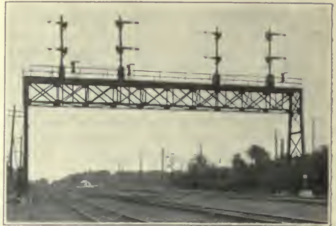
FIG. 287. SIGNALS. Standard signal bridge on the Illinois Central Railroad near Riverdale.
